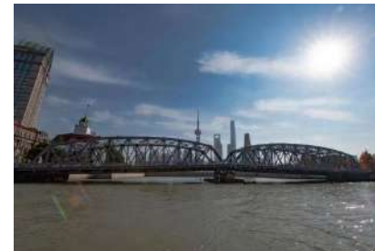
Waibaidu Bridge after historical subsidence
