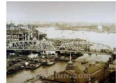
Waibaidu Bridge before historical subsidence
