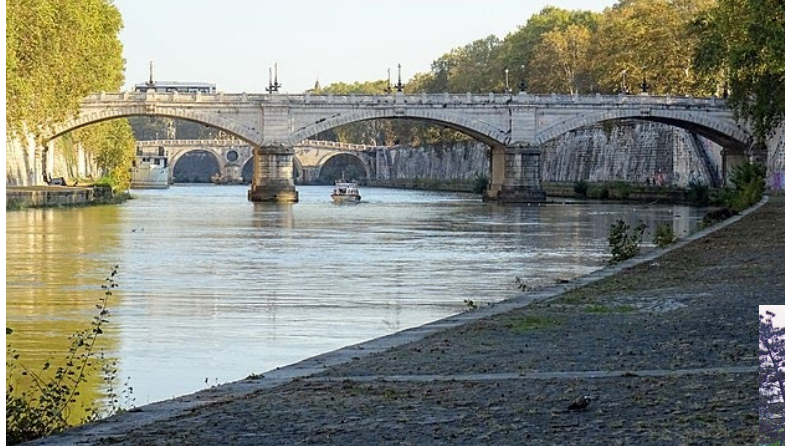
Arc bridges across the Tiber River, Rome
